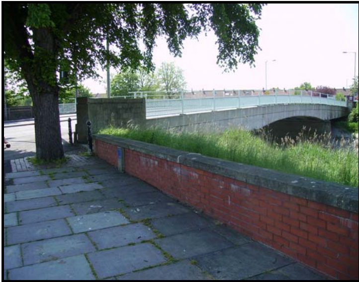
Bridge and Flood wall
