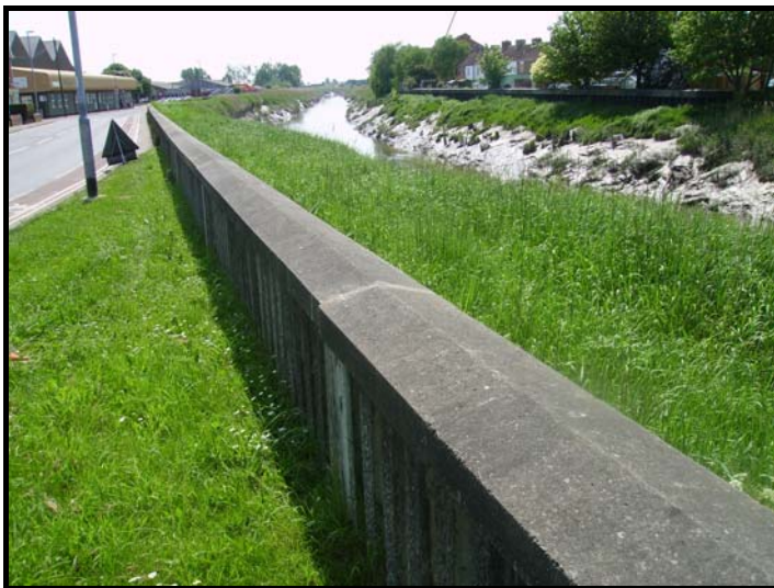
Concrete Flood wall
